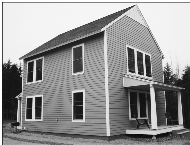
Judith Cullen and her family moved into one of the first two houses finished at Ripples Hill. Construction of a third family’s house may begin this spring.
